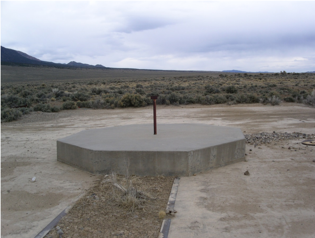
Figure A-1. Photo Showing the Concrete Cap that Covers the UC-3 Emplacement Borehole
