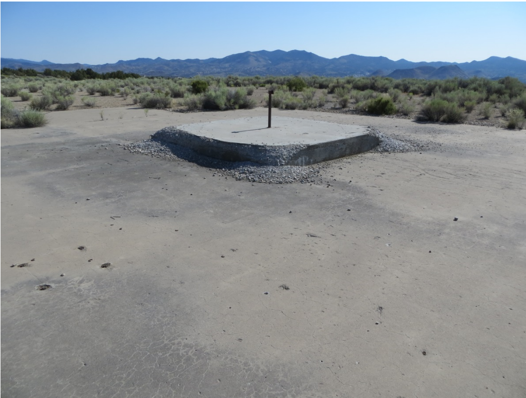
Figure A-2. Photo Showing the Concrete Cap that Covers the UC-4 Emplacement Borehole
