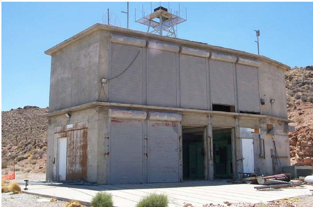
Figure A-22. Building 400, a camera station for photographing atmospheric tests, at Area 6 Control Point built in 1951 and demolished in 2003. One of the first buildings constructed on the NTS to support weapons testing activities (2003 Photo).
