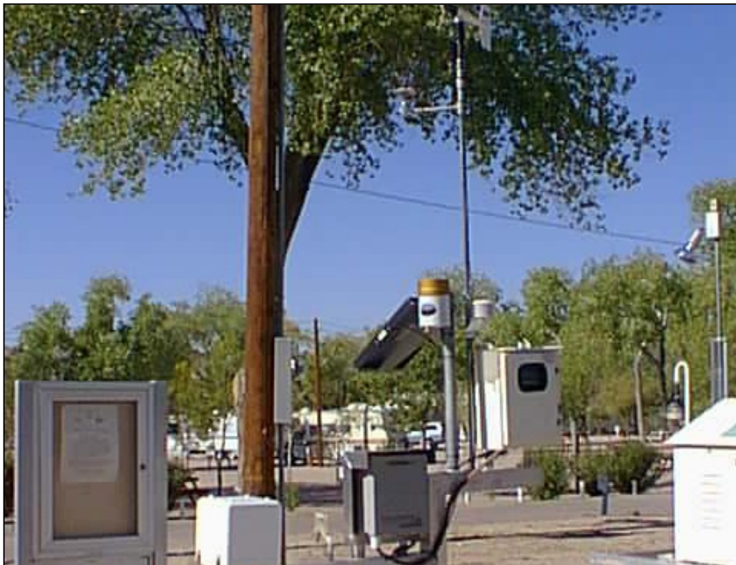
Figure 5-2. CEMP station at Beatty, Nevada
