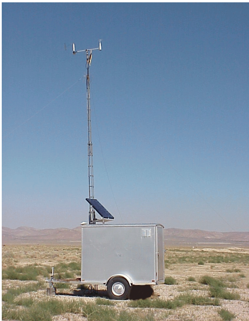
Figure 15-1. Example of a typical MEDA station with 10 meter tower
