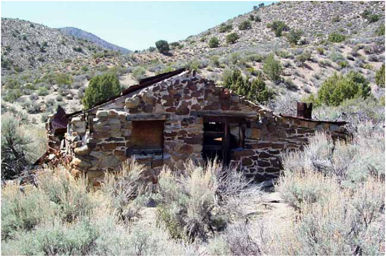
Figure A-23. Bower cabin on the NTS (photo by DRI, 2001)
