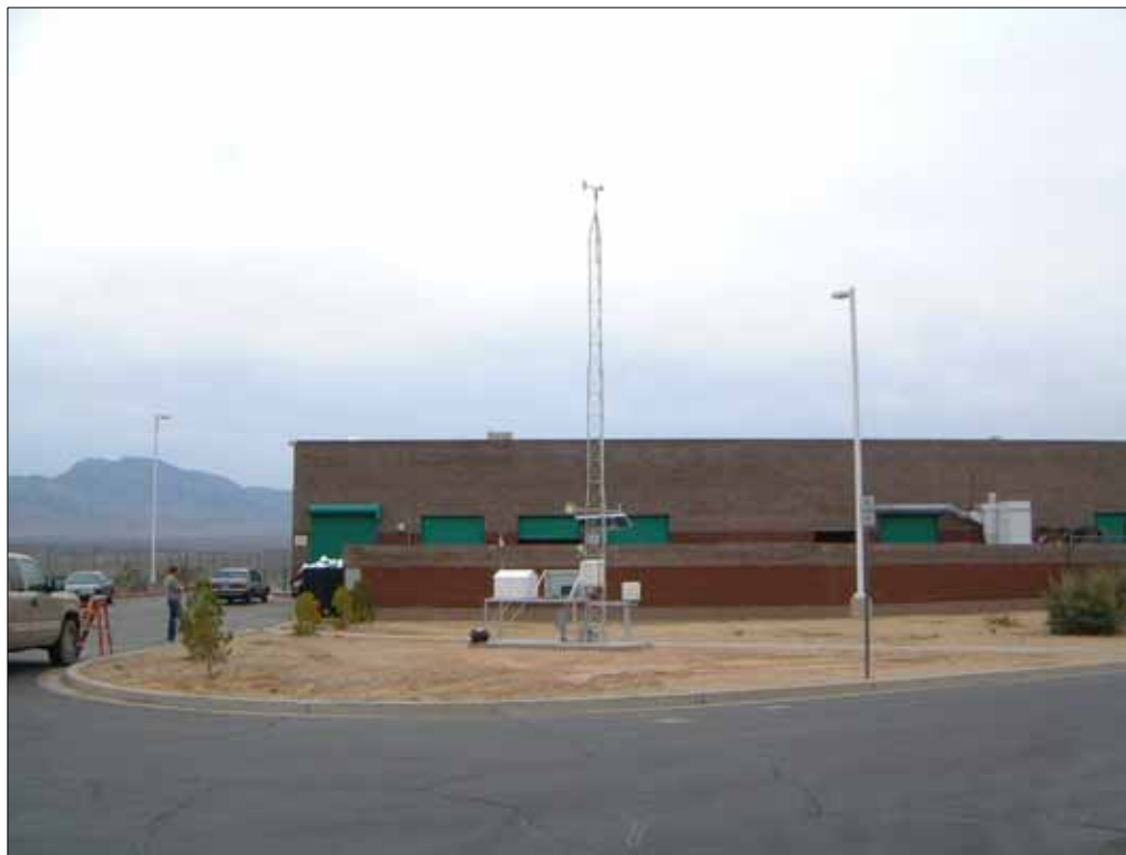
Figure 6-2. CEMP station at Mesquite, Nevada
