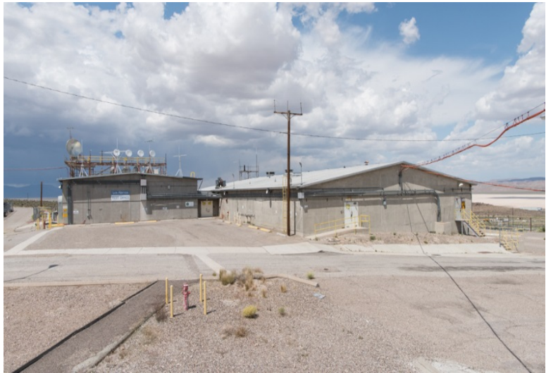
Figure 12-1. Control Point Building CP-1
