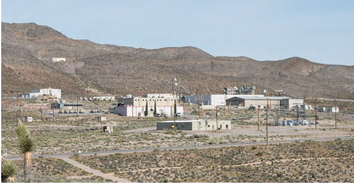
Figure 12-1. Overview of the Area 6 Control Point Facility (Remote Sensing Laboratory 2016)
