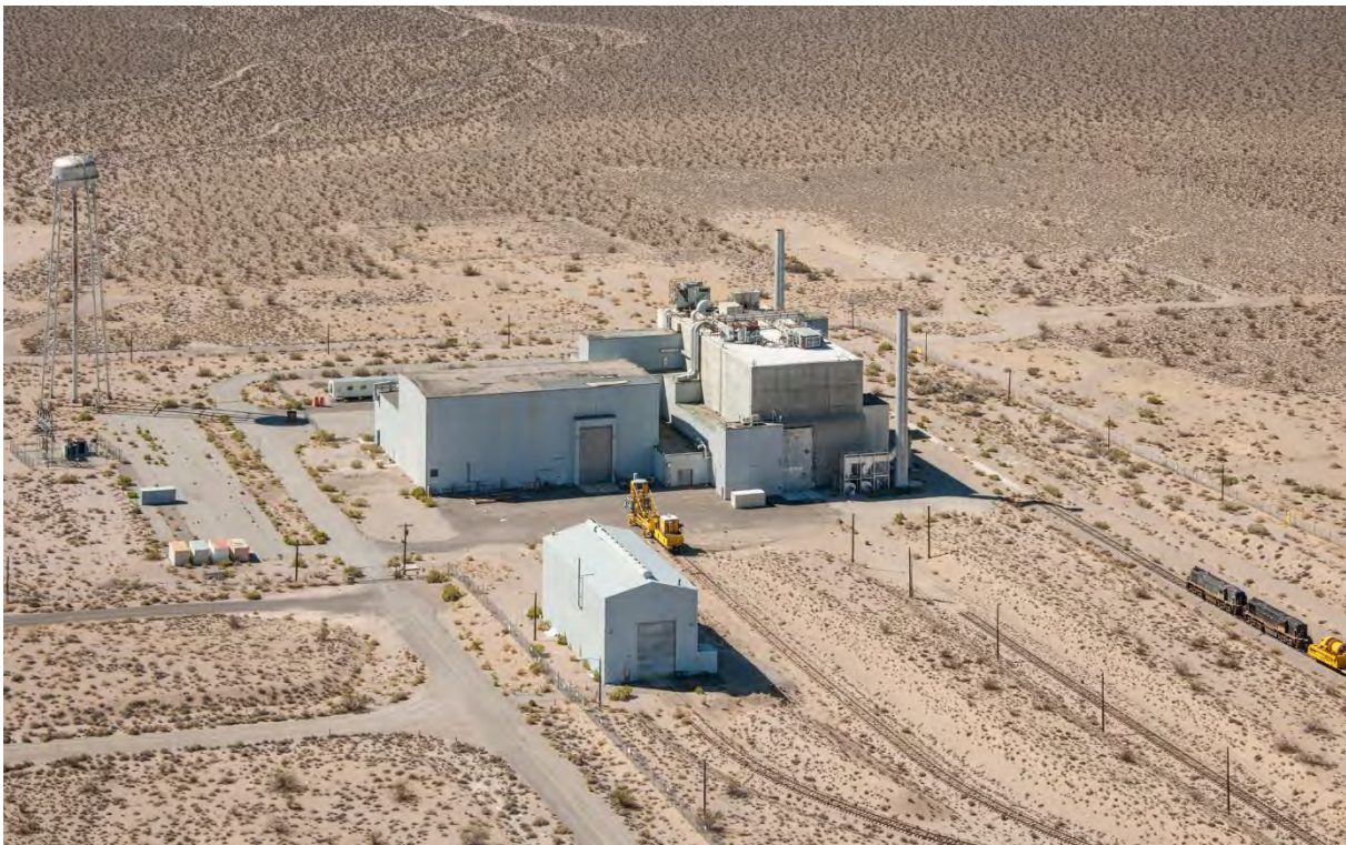
Figure A-27. The NRDS Engine Maintenance and Disassembly Building (photo taken by Remote Sensing Laboratory 2013)
