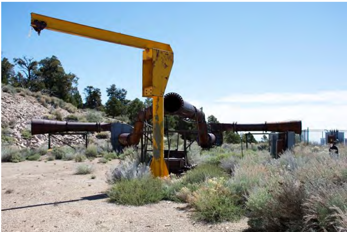
Figure 12-4. Overview of the U12n.10 Vent Hole System (DRI 2020)
