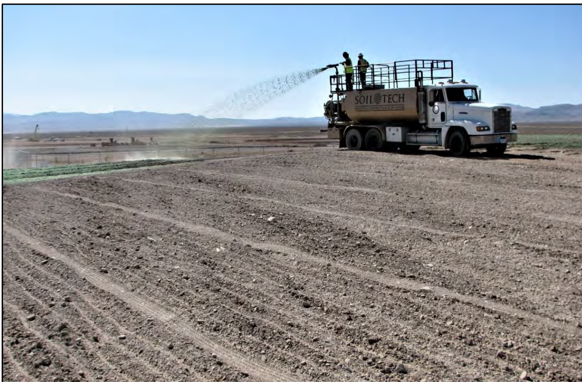
Figure 13-7. Applying hydromulch at the Cell 18 Cover Cap (Photo by D.B. Hall, October 26, 2020)
