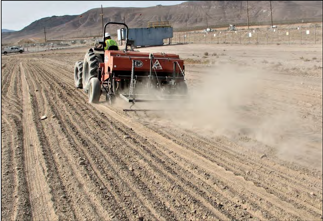
Figure 13-6. Seeding Cell 18 Cover Cap with chain harrow to cover the seed (Photo by D.B. Hall, October 22, 2020)
