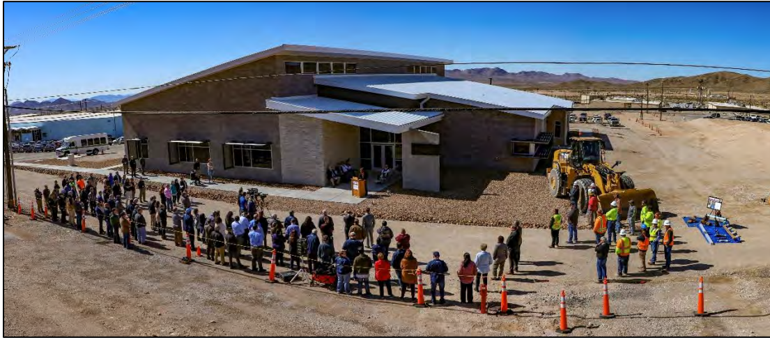
Figure 3-1. Mercury Modernization Building 1, 23-460
